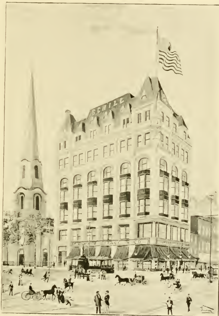
U. S. CREDIT SYSTEM COMPANY'S BUILDING.
